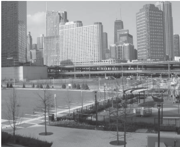
Figure 4: Sectional condition at Lake Shore East; all three levels of Wacker Drive are visible in the background.
