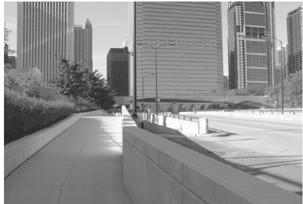
Figure 3: Sectional condition where slip ramps emerge from underground parking at Millennium Park, Chicago, IL.
