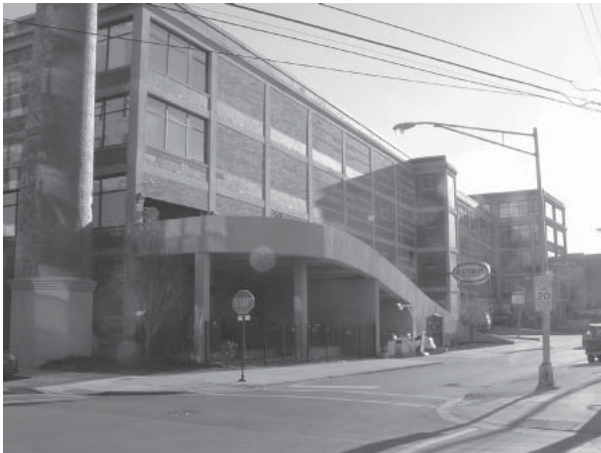
Figure 5: Ramp to embedded parking at Trader Joe's, North and Clybourn, Chicago, IL.
